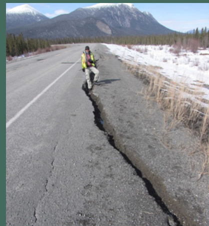
Figure 2. Tarmac road crumbling due to permafrost thaw (Dore, 2021).
